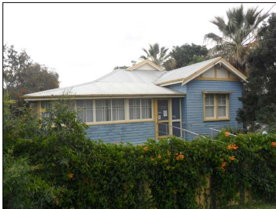
Plate 3 – Existing structure proposed for café/restaurant use on Lot 3 DP 337280
